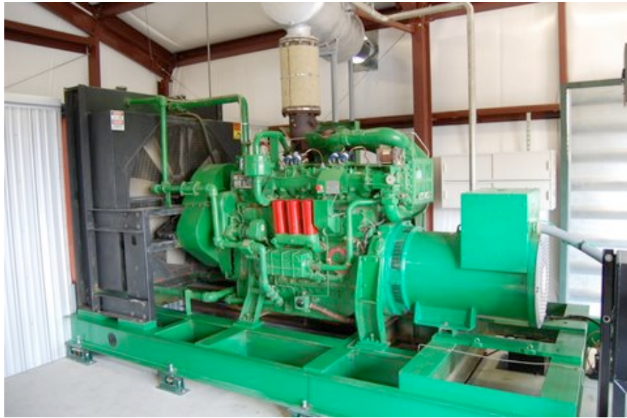
Figure 3. GkW Energy's Waukesha Engine-Gen Set (Cox, 2011)
